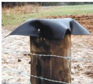
To preserve wooden posts, William Johnson simply nails a section of rubber belting on top to keep rain off.
