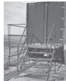
They added steps, railing, and unloading platform on back.
