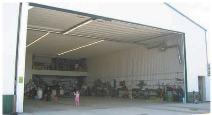
When support post is rolled to the side it creates a 40-ft. wide opening.
