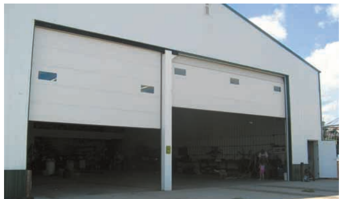
The Richters' 54 by 80-ft. shop has a 16-ft. door and a 24-ft. door with a moveable post in between.
