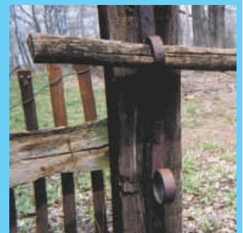
Metal rings make it easy to hang rails on posts. A single nail holds rail in place.
