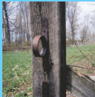
Metal rings make it easy to hang rails on posts. A single nail holds rail in place.
