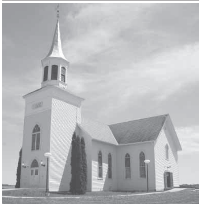
The Lindquists paid movers $80,000 to move the 60 by 80-ft. building 1/2 mile down the highway. "It was worth it because it's good for the community," they say.
