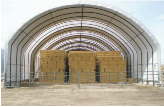
By developing a system to bend oilfield tubing, Jim Klys and Richard Schmidt came up with a system to construct their own canvas-covered hay sheds and storage buildings.
