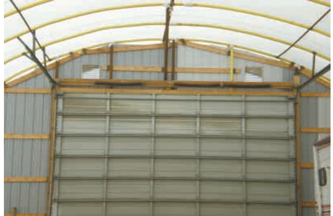
To make shed's arches, the men pound a half-moon pattern of steel fence posts into the ground, then use a tractor to bend tubing around the half circle.
