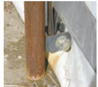
Ratchets fitted with seat belt straps are welded to the bottom of uprights to hold canvas snug.
