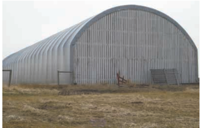
End walls of hay sheds are covered with slatted wood to increase air circulation. On other buildings, the ends are closed in completely with either tarp, tin or wood.
