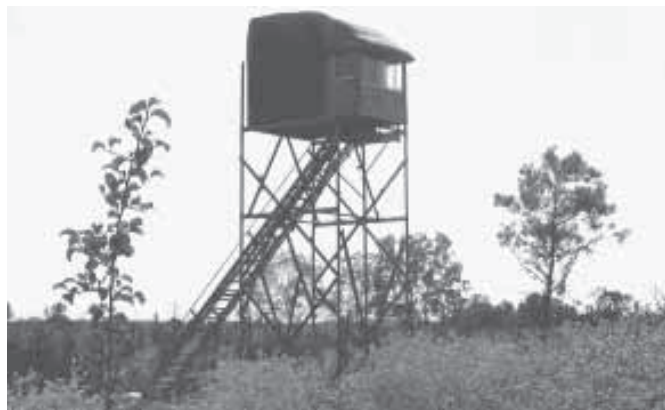
"It provides a comfortable place to see wildlife," says Chuck Braddock, who built this deer stand from a semi tractor's sleeper cab, adding stairs made from conveyor parts.
