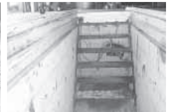
Door opener moves 10 4-ft. cover sections of 1/4-in. thick deck plate back and forth across top of pit. When rolling oil pan is full, Dorwin moves it to the end of the pit to dump.
