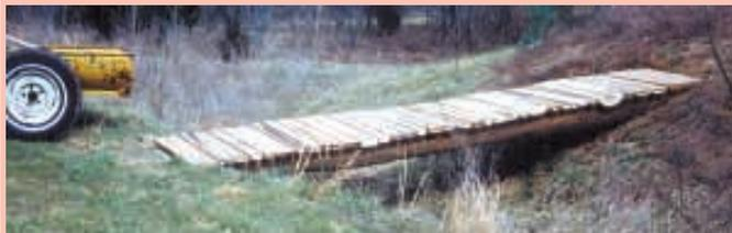
Bill Reeks made this "mini bridge" by cutting an electric pole in half and adding a deck made from scrap 2-in. lumber.
