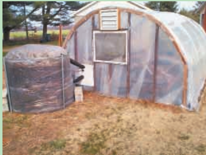
To supply heat, Katherine Brooks ran pipe through a 5-ft. dia. compost pile at one end of her greenhouse. Compost pile is contained by a wire mesh frame.
