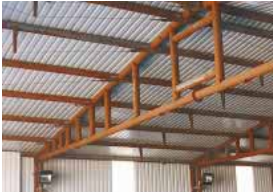
Kroenlein uses 6 or 6 5/8-in. dia. steel pipe for trusses, sidewall framing.
