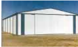
Buildings are as big as 80 ft. wide and 150 ft. long. This 60 by 120-ft. machine shed has an 18-ft. eave and 17-ft. high, 30-ft. wide double sliding doors.
