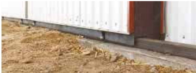
Sliding doors have bearings along the bottom that run against a guide. Bearings are self-cleaning and don't retain water so they won't seize up in cold weather.
