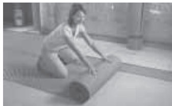
Plastic floor pad is dimpled to create 5/16-in. air gaps between the concrete and the wood or carpet flooring surface. Keeps flooring from direct contact with concrete, preventing wicking of moisture.
