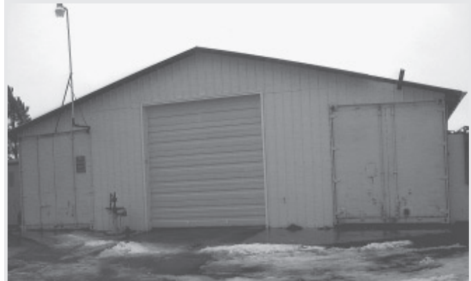
Schuster built a shop between two 40-ft. containers, which form the building's walls.
