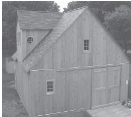
Kit uses pre-cut and drilled lumber and hardware. No prior building experience is required to erect a building.
