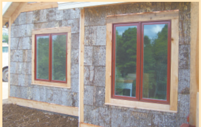
A North Carolina company sells poplar bark siding made from Tulip Poplar trees harvested in the Appalachian Mountains.
