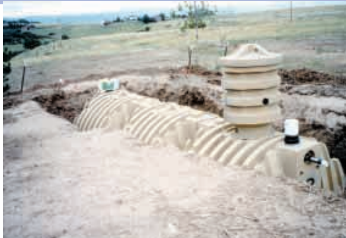
Darco's 2,000-gal. poly storage tanks are designed for use underground.
