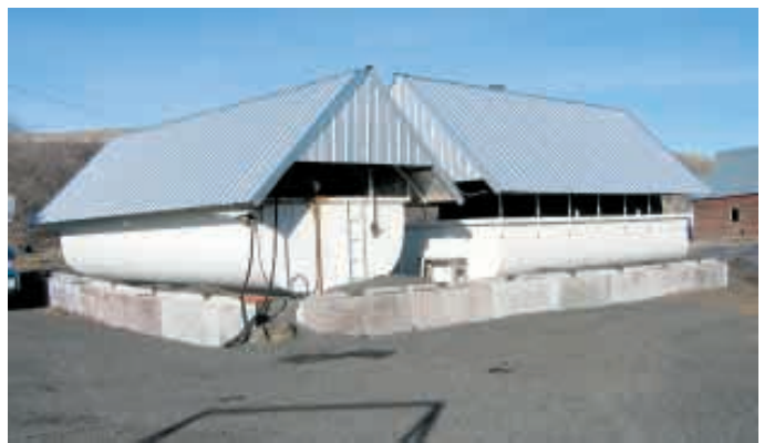
Mark Richter built two 10,000-gal. fuel containment structures and covered them with a metal roof to shade the tanks and keep rain off them.
