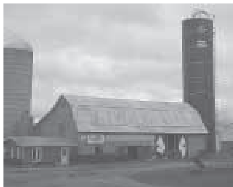
A pair of Canadian-based companies buy and sell second hand Harvestore silos, transforming them into top unloading silos.
