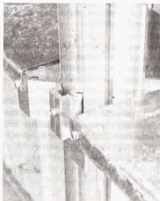
Adjustable brackets bolt to the aluminum "studs".
