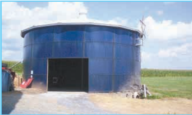
Karl Herr no longer needed his 42-ft. dia. Harvestore Slurrystore, so he put a roof on it and cut a big door into the side to convert it to a hay shed.
