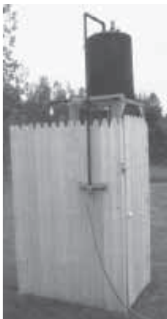
Outside shower hooks up to a garden hose and uses sunshine to heat the water. A water heater, painted flat black, mounts on top of wood frame adjacent to shower stall.
