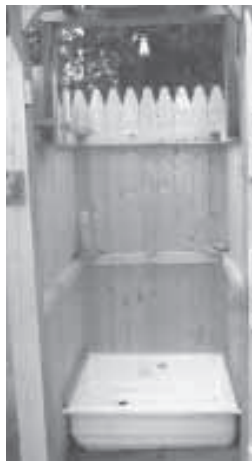
Outside shower hooks up to a garden hose and uses sunshine to heat the water. A water heater, painted flat black, mounts on top of wood frame adjacent to shower stall.
