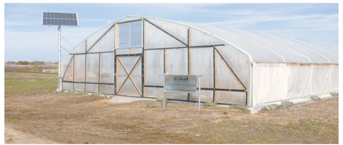
Solar panels on Four Season's moveable high tunnel greenhouse power thermal-controlled side panels and roof peak vents.
