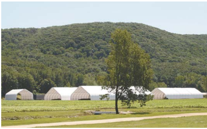
To avoid spreading raw manure on fields, Laurelbrook Farms started composting. After two years they put up these hoop-type buildings.
