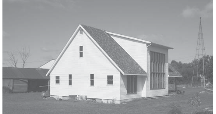
He wanted a cathedral ceiling in the living room area so he added a dormer with a glass front on one side.
