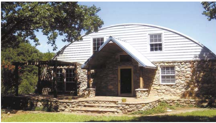
Yvonne and Patrick Taylor converted half their 45 by 72-ft. Quonset building to living quarters. Photo shows front entry.
