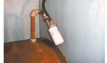
About 30 ft. of service station hose runs from the pump to a waste oil tank in another room, where oil runs through a filter mounted above tank.
