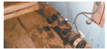
About 30 ft. of service station hose runs from the pump to a waste oil tank in another room, where oil runs through a filter mounted above tank.
