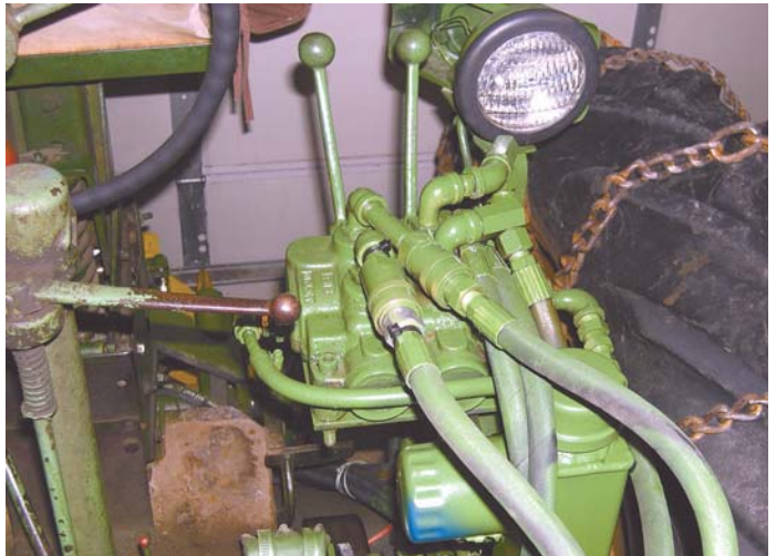
Bipes welded up brackets to bolt on a hydraulic pump and valve.
