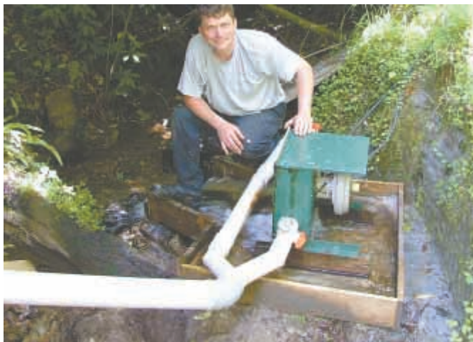
Even a small amount of water is enough to activate the micro hydro Pelton turbine. It concentrates small flows under high pressure through jets inside a sealed box.
