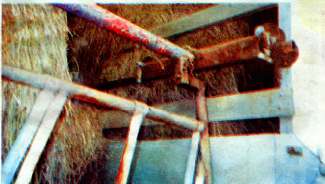
Gates ride on pipe rails mounted above 4-ft. high concrete sidewalls. Gate hinges on roller bracket so either end of gate can move forward without damage to end of gate.
