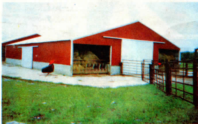
There's a feed gate at each corner of Wood's 62 by 96-ft. self-feed bale barn. Bales are stored down the center and loaded into feed alleys on either side of building as needed.
