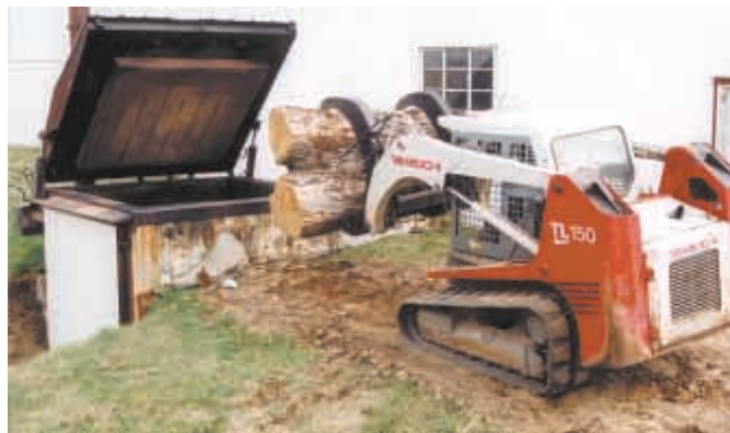
They use a skid steer with a grapple to load up to three 6-ft. logs at a time.
