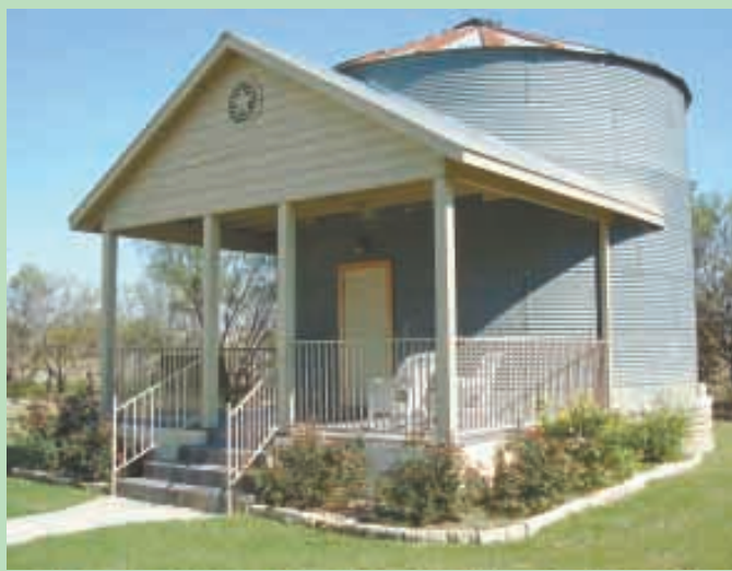
One-of-a-kind home is built from a 1940's 20-ft. dia. grain bin. The large, covered front porch is surrounded by beautiful landscaping.
