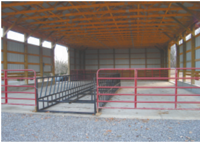
When Eric Blanford built a 40 by 80-ft. building for his cows, he installed a 30-ft. long, 6 1/2-ft. wide bunk down center of building. He fills it by pushing bales into the open end.
