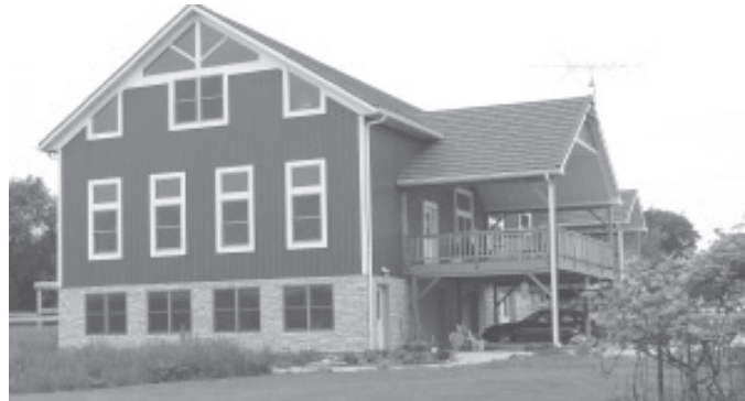
"There was already a loft over grain bins at one end of barn. I added a loft at the other end over my bedroom," says Shari.
