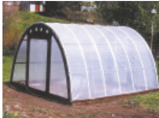
Day made the end caps out of wafer board by bending a piece of pipe into a half circle and laying it across three 4 by 8 sheets, which he cut into an arc.
