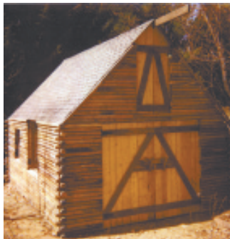
Pressure-treated landscaping ties, found behind an electrical cable company, were used to make cabin's walls.
