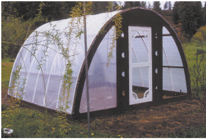
What makes Harry Day's greenhouse different is the strength of wood and the way he attaches 20-ft. long, 3/4-in. dia. pvc "hoops" to the 2 by 6's that run down each side.
