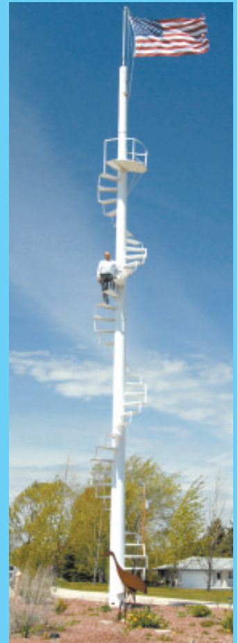
Jim Kocourek's 57-ft. flagpole started out as a 100-ft. radio tower used to dispatch service trucks at a Deere dealership.
