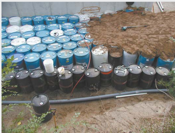
Erickson buried 320 barrels filled with water to store heat from greenhouse.
