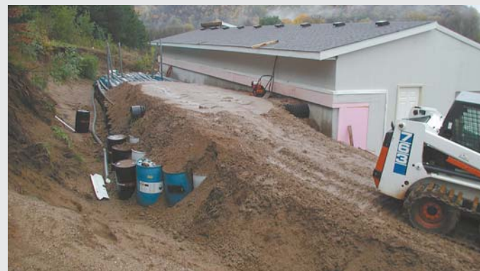
Double layers of insulation were laid over and under heat storage barrels before they were covered with a thick layer of dirt.
