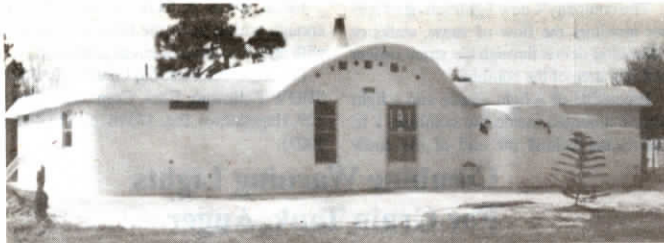
The frame of the concrete house was formed with more than 16,000 ft. of 3/8-in. dia. steel reinforcing rod.
