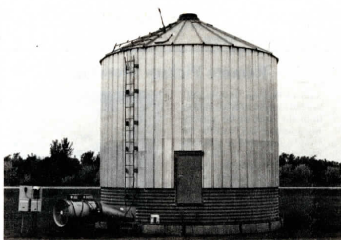
Liner insulates outside walls of drying bin and draws moisture out.
