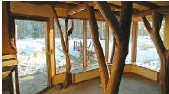
Whole Tree Architecture uses tree trunks for everything from structural components (above) to interior decorating, including stairs, railings and exposed columns.
