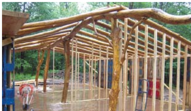
Whole Tree Architecture uses tree trunks for everything from structural components (above) to interior decorating, including stairs, railings and exposed columns.
