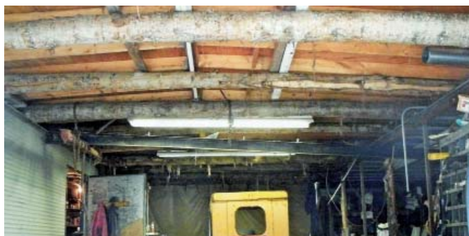
The Sextons used hoists to set "whole tree rafters" in place.
