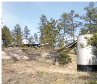
Water drains out of trampoline and is piped into a 7,000-gal. storage tank (left). Tarp stretches across a round metal frame. Note metal drain in ground (right).
