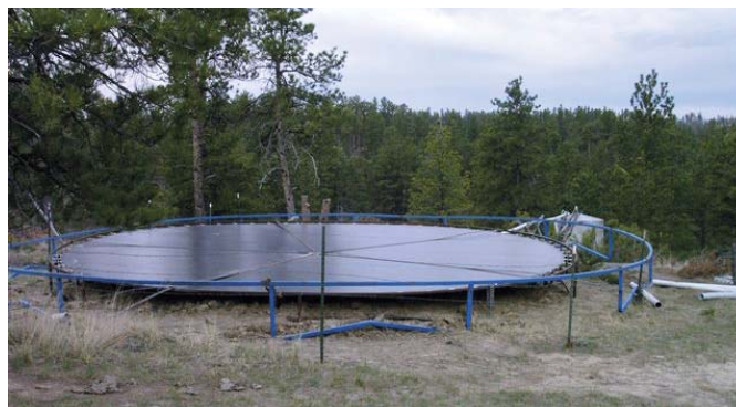
Giant poly “trampoline” catches rainfall in remote pastures and stores it.
