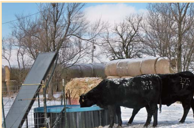
A 4 by 8-ft. solar panel sets outside tank, with a small pump circulating antifreeze from panel to a copper heating coil inside pvc drinking tube.
