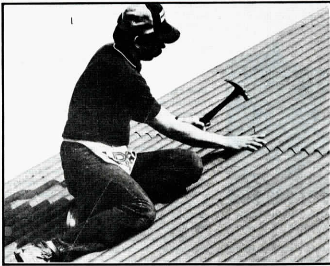
Asphalt roofing sheets are available in 8 colors with smooth or granulated finish.
