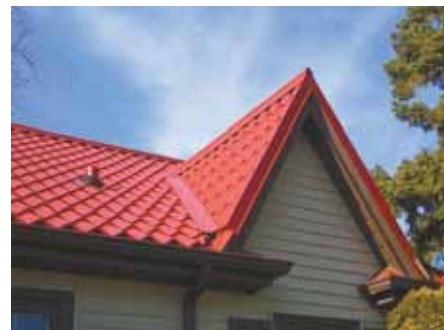
Met-Tile resembles clay tile yet weighs just 125 lbs. per square (1.25 lbs. per sq. ft.).
