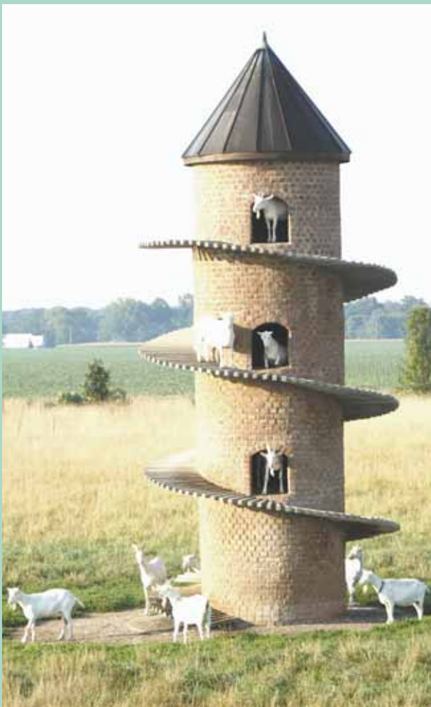
Goats stay fit and entertained climbing this 31-ft.tall “goat tower”. It has 276 concrete steps, arranged in a spiral pattern.
