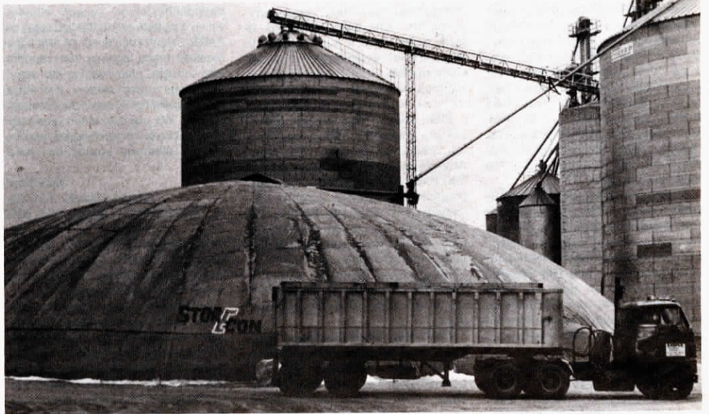
Forced air keeps dome inflated while being loaded or unloaded, and helps aerate grain.
