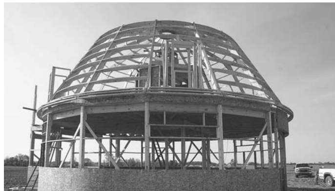
He built the structure like a pole barn, starting with a center point and a 20-ft. board to mark where to place the laminated 2 by 6 posts for the 40-ft. dia. building.
