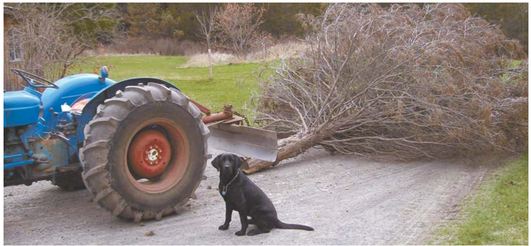
Frank Taylor came up with a simple way to do a better job grading his driveway – he drags a big Juniper tree behind the tractor with a chain. Tree spreads gravel dug up by the blade and fills the potholes.
