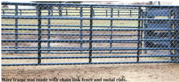
Wire frame was made with chain link fence and metal rods.
