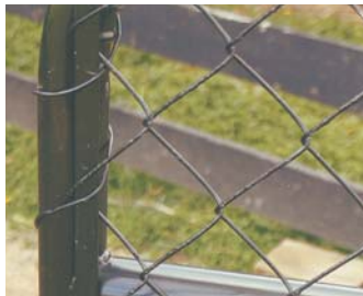
Close-up photo shows how wire is tied to gate.
