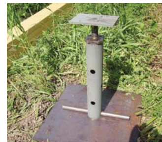
To raise the cabin, Dupont hooks up hydraulic jacks to telescopic metal posts.
