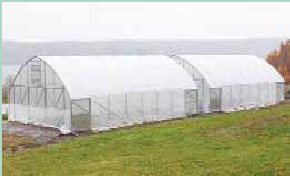
Two 30 by 48 three-position movable greenhouses on V-Track, photo courtesy of Wegman's Food Markets, N.Y.
