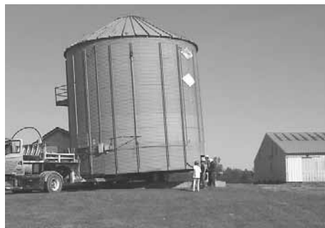
Bruellman and crew pull a 36-ft. dia., 31-ft. high bin over a bridge (left). Top dryer bins are movable, too (below).
