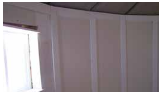
To build the loft Thiebes used 2 by 10-in. floor joists, which are supported by triple 2 by 4’s nailed together to make posts (above). Wood strips cover the joints between sheets of drywall.
