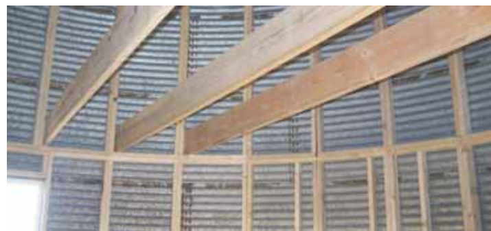
To build the loft Thiebes used 2 by 10-in. floor joists, which are supported by triple 2 by 4’s nailed together to make posts (above). Wood strips cover the joints between sheets of drywall.
