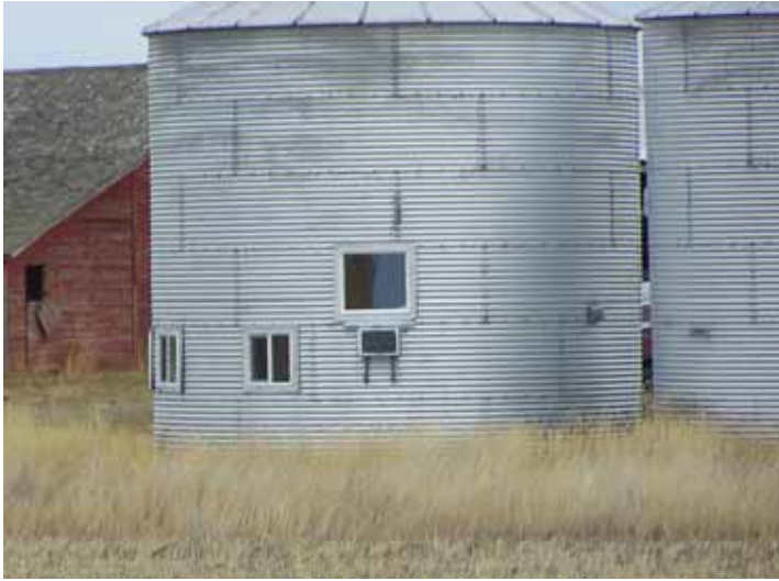
Soon after he bought a farm in central Montana, John Thiebes built living quarters inside this unused 18-ft. dia., 2,800-bu. grain bin.
