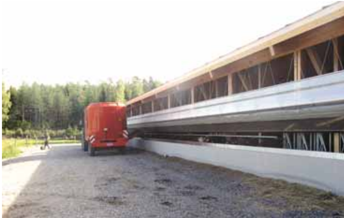
Finnish design allows feed bunks to be filled from outside of barns.
