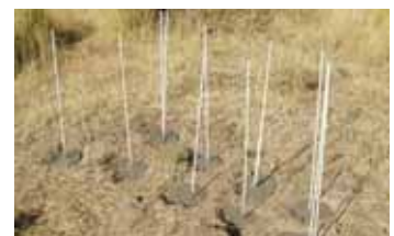
Fence post “doughnuts” are blobs of concrete with a hole in them that supports the post.
